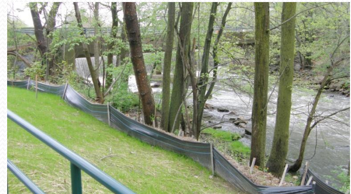
Careful Erosion Control and Bank treatments
