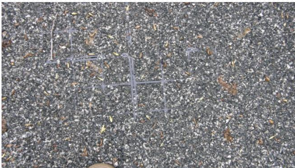
Fully Permeable, Grid Reinforced, Stone Dust Trails
