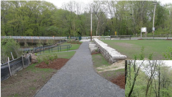
Fully Permeable, Grid Reinforced, Stone Dust Trails
