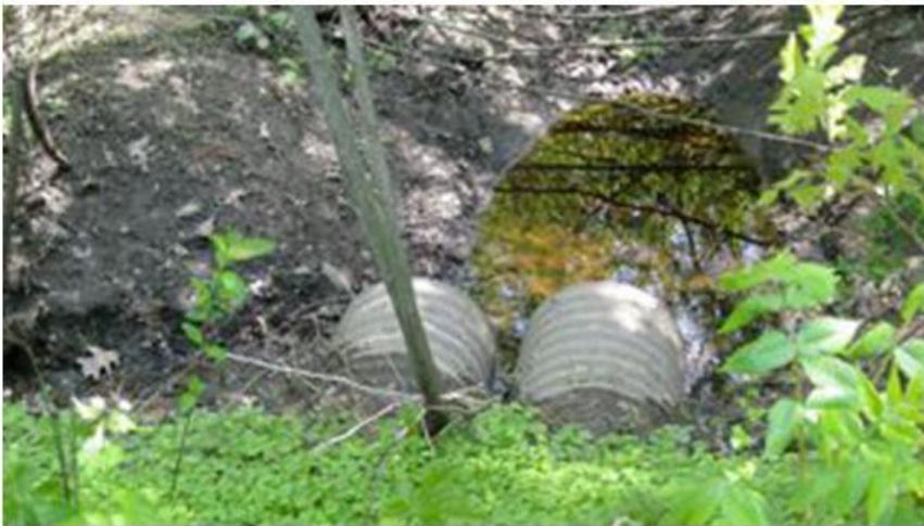
Silted up concrete pipes
