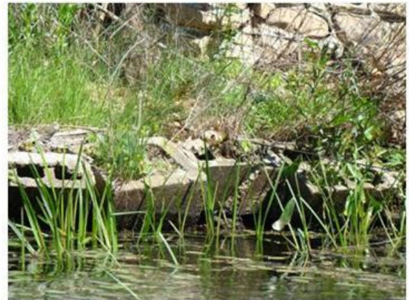
Close up of failed retaining wall
