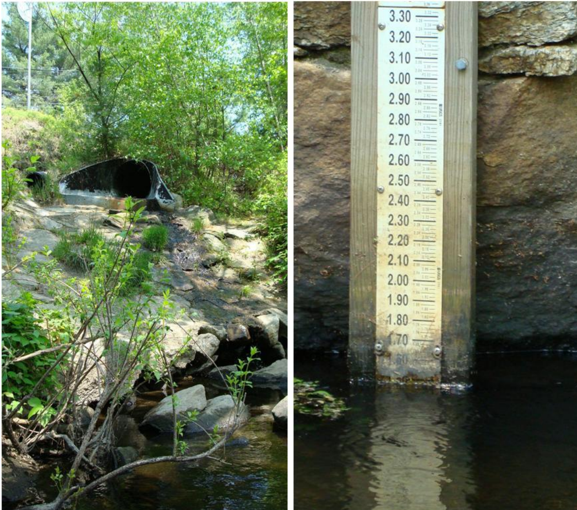
Pleasant Street Bridge – (left) drain pipe has dry weather discharge (right) water depth at time of survey
