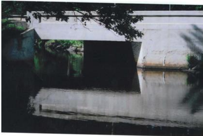
Wheeler Road Bridge
