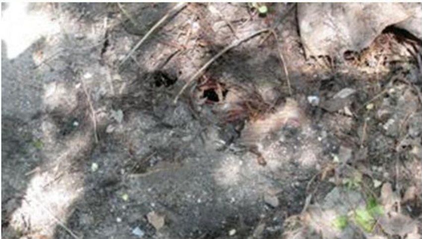
Clogged drain Route 140
